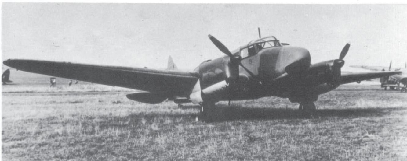
AS504 was the sole Oxford fitted with Gipsy Queen IV engines. This photograph is of interest in that, when it was released publicly during the war it "leaked" the Mosquito, whose tail can be seen under the starboard wingtip and which, at that time, was still secret.
